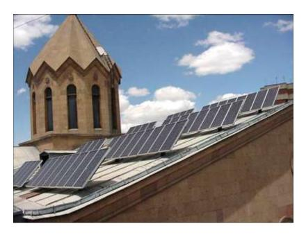
$Solar\ photovoltaic\ panels\ at\ the\ roof\ of\ Surb\ Sargis\ church\ in\ Yerevan$
