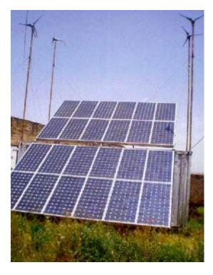
Fig. 6.14. Combined system of solar photovoltaic panels and wind turbines
