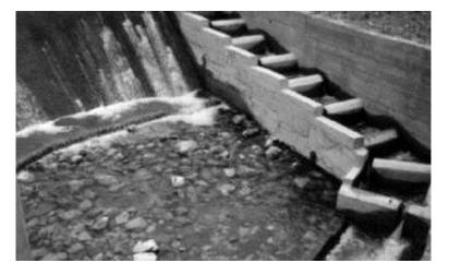
Fig. 10.12 Fishpass with vertical slots [52]
