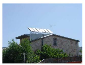
Fig. 6.12. Solar water heating system. Total area of solar collectors is 13m2 (2006)
