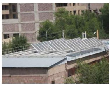
Fig. 6.11. Solar water heating system integrated with boiler house. Total area of collectors is  $70 \text{ m}^2$  (2008)
