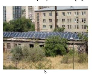
Fig. 6.10. Solar water heaters: a. Solar water heaters at the roof of Red Cross Rehabilitation Center (Yerevan); b. Solar water heaters at Narcologic Clinic integrated with back up gas boiler (Yerevan)
