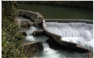
Fig. 10.11 Fish pass of rustic construction [52]
