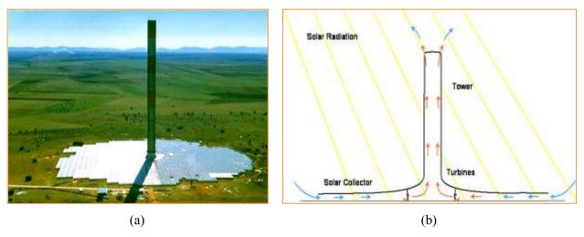
Fig. 4.7. Solar chimney in Manzanares Spain: a) Common view, b) The scheme of operation of Solar chimney
