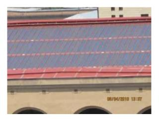
Fig. 6.9. 10 kW solar photovoltaic station installed at Armenian-American Health Center
