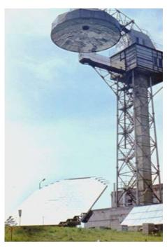
In 1984, a unique solar furnace with 10m diameter parabolic concentrator with vertical optical axis, 120m² surface area, sun tracking heliostat and 1.2 kW off-grid PV station have been commissioned. The installation had been designed for material science needs and, in addition, had a cylindrical thermo-PV receiver placed in the focus of the parabolic mirror concentrator.
