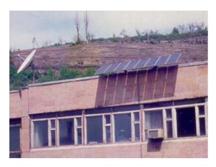
Solar photovoltaic panels at the roof of SEUA
