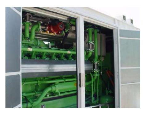
Fig. 7.6. Gas engine installed at Lusakert Biogas Plant
