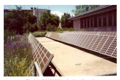
Fig. 6.4. 7.5 kW PV station in t. Gyumri
