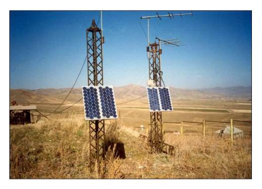
PV systems to provide seismic observation stations with electricity
