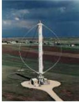
Fig. 8.3. Vertical axis wind turbine
