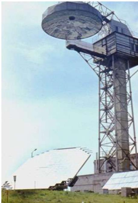
In 1984, a unique solar furnace with 10m diameter parabolic concentrator with vertical optical axis, 120m<sup>2</sup> surface area, sun tracking heliostat and 1.2 kW off-grid PV station have been commissioned. The installation had been designed for material science needs and, in addition, had a cylindrical thermo-PV receiver placed in the focus of the parabolic mirror concentrator.
